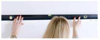
Place the top track at desired height, mark one hole in the middle.
