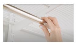
3. Mount the rod into the rod holders. First, snap joining rods into a closet rod holder and second, snap the outer end of each rod into the outer closet rod holders.
